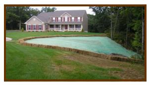
The use of erosion matting for slope protection provides successful erosion control and prevention of sedimentation to the adjoining woodland.
